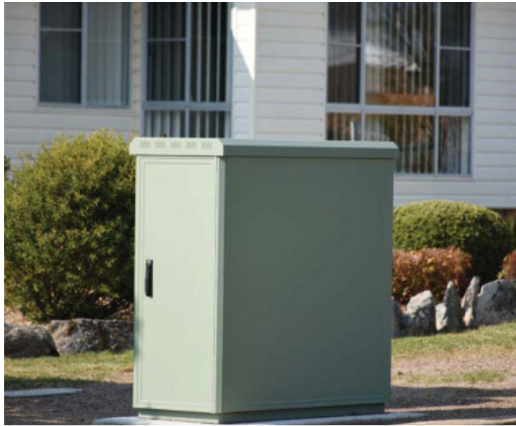
Guyra will be serviced by both Fibre to the Node (seen here in Wirruna St) and Fibre to the Curb
