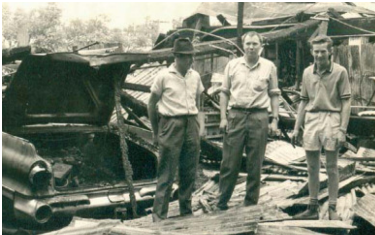
On November 30, 1967 Burgess Garage burnt to the ground. The Guyra Guardian reported that 'the fire was one of the worst in the living memory of Guyra residents and may have caused damage up to $50,000.' The fire was caused by an accident with thinners and a welding spark. Pictured above in the ruins of the building are Des Mulligan, Brian Vickery and Don Williams.
