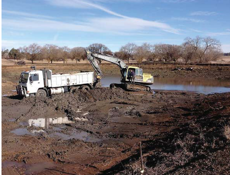
DIRTY WORK: Cleaning out the 10th dam at the golf course. The dam is already full again after the recent rain
