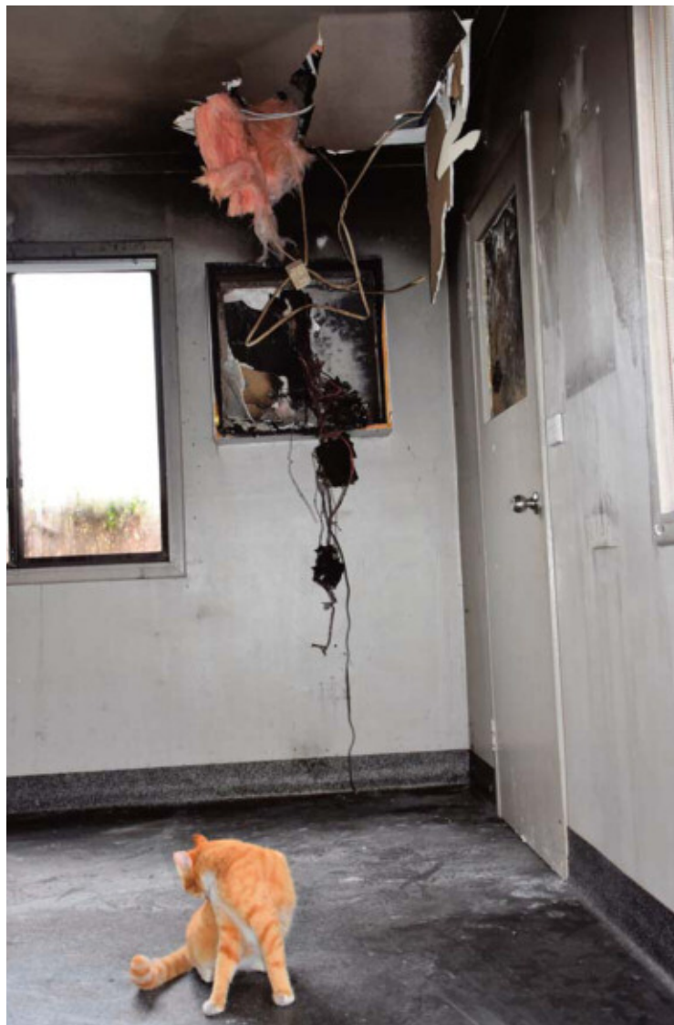
Fire began in the electrical switchboard
