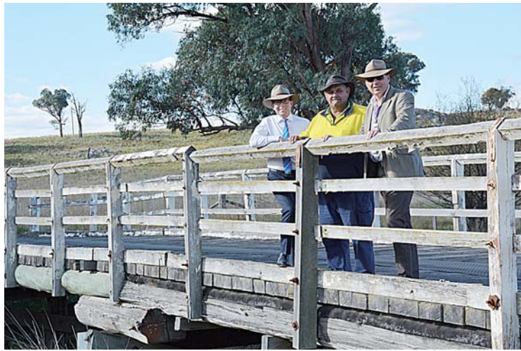
Northern Tablelands MP Adam Marshall, left, with Armidale Regional Council's John McLeod and Mark Piorkowski on Laura Creek Bridge near Guyra, one of the ageing timber bridges slated for replacement.
