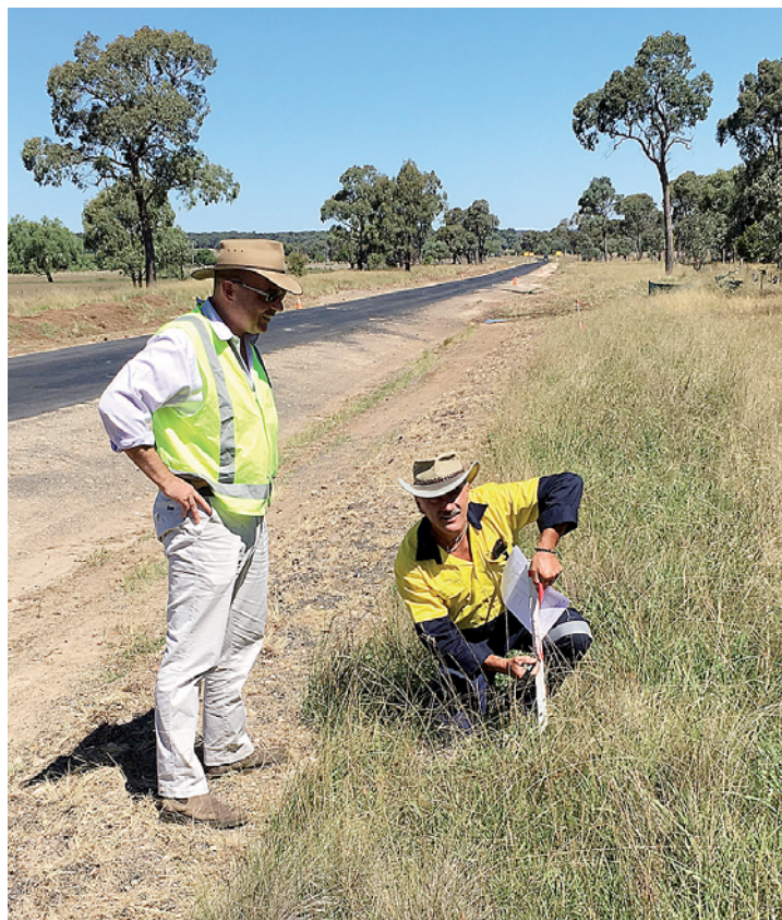
Armidale Regional Council's Group Leader for Service Delivery, Mark Piorkowski, and Works Overseer, Paul Little, inspecting the Guyra-Tingha Road works site.
