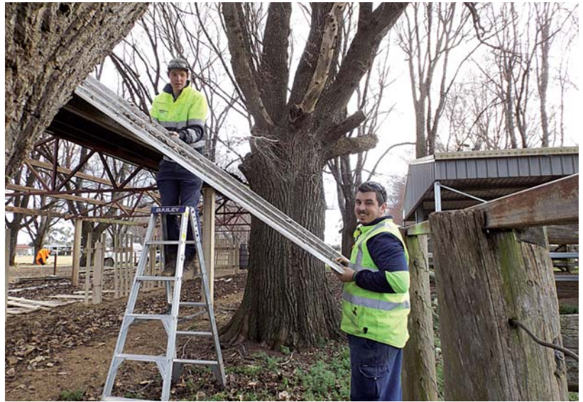
Demolition in progress - Dean Field and Cowin Campbell
