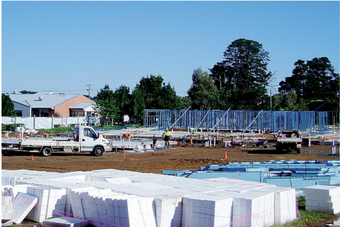
The new aged care facility is taking shape and should be completed by the end of September
